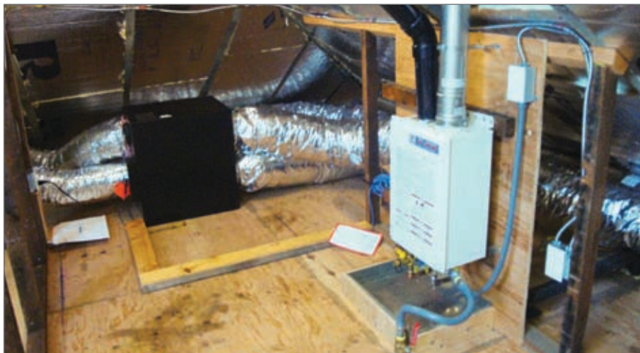
An energy recovery ventilator with ductwork is installed in the attic. Whatever heat is generated by daily activities is returned to the house. A Takagi instantaneous water heater is on the right in the photo.
